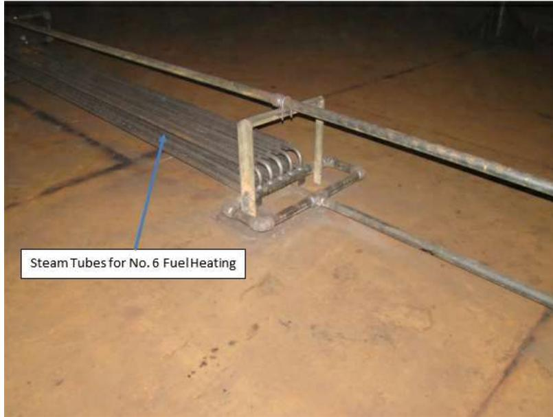
Figure 3: Tank 2 Platform Heater
