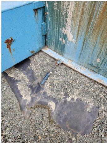
Figure 15: View of grounding cable.
