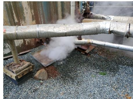
Figure 8: View of drip pans in place to protect liner.
